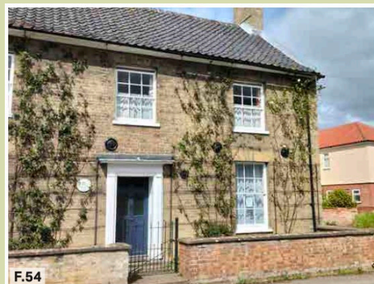
Figure 54: Photo of a 2 storey dwelling in Chedgrave.
